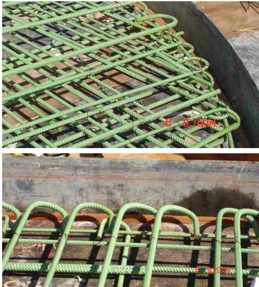
Figure 1.1. Construction photos 1 of tilted reinforcing hooked bars
